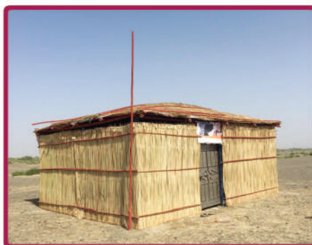
Pic 3: TLC Built by OSDI in Danok
