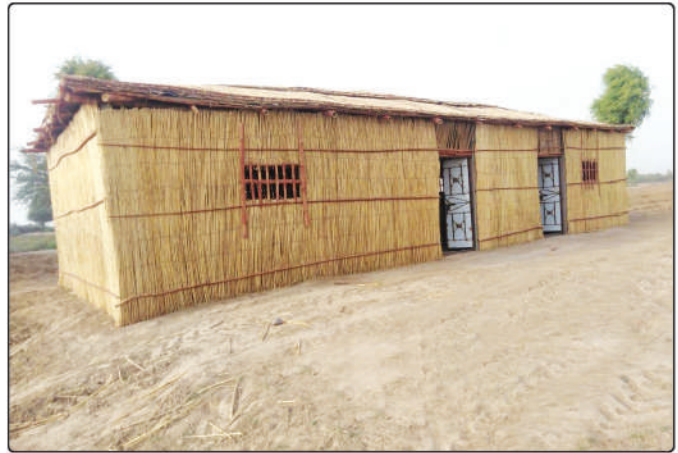
Two Classrooms based TLC constructed by OSDI in Sayarani Goth
