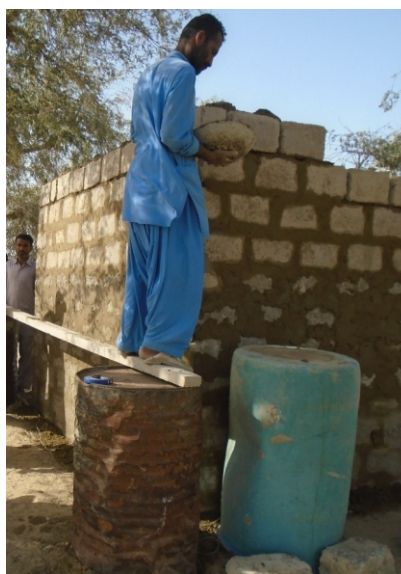
Picture 23: Construction of cemented water base in Bohaar (Moosa Goth)
